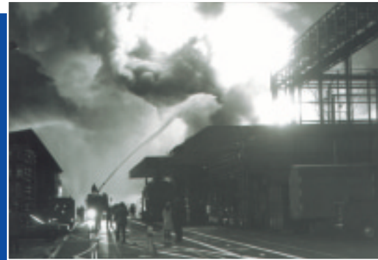
Sandoz warehouse fire, 1986
