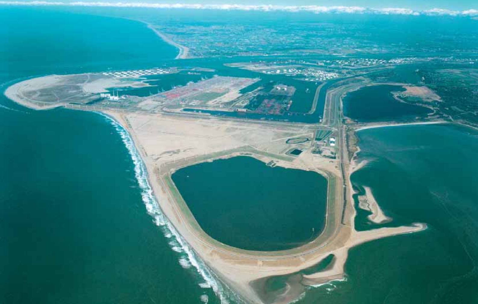
Depot "de Slufter" in Rotterdam
