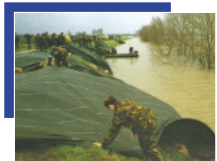
Flood fighting: shielding an embankment
