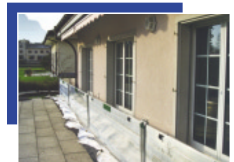
Sealing the shell of buildings (mobile)
