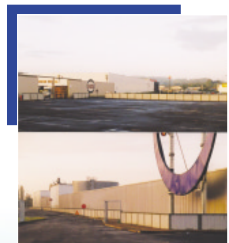
Flood wall shielding (Meuse, F)
