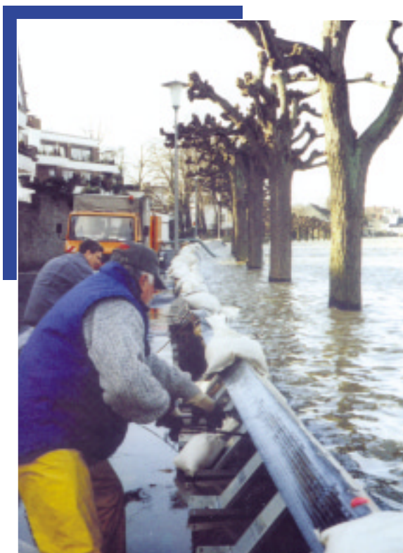
Raising protection barriers (mobile)
