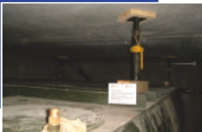
Oil tank protection against buoyancy (Basel)
