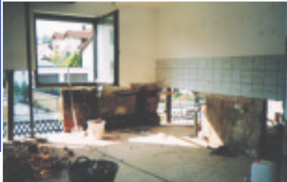
Replacing brickwork following oil pollution in Neustadt / Donau (Kelheim district) 1999
