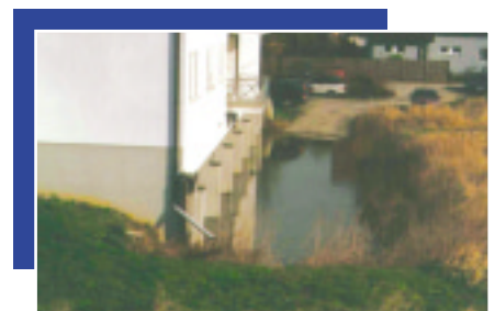
Rise of groundwater
