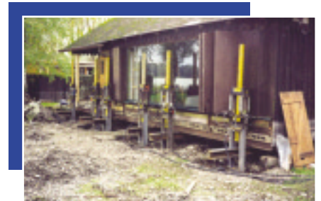
Elevating light constructions
