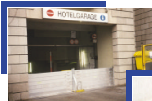
Sealing openings (mobile)
